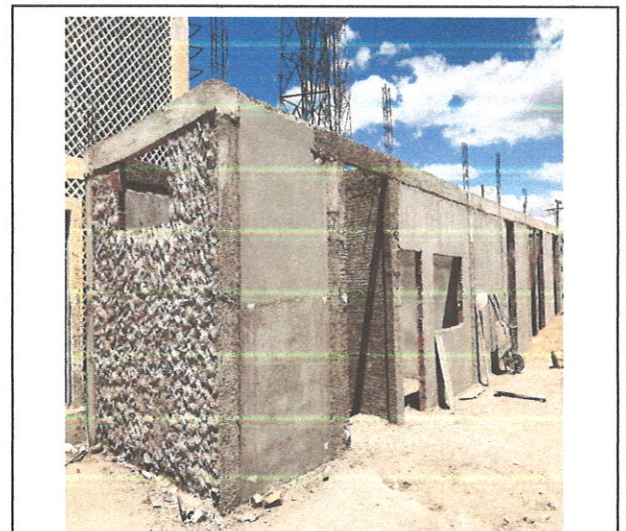
FOTO 72: Reboco (bloco 3)
